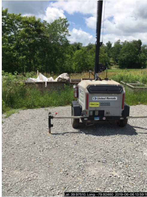
Photo # 11. Additional refuse bags and a generator powered light were also noted in the south west corner of the pad without containment.
