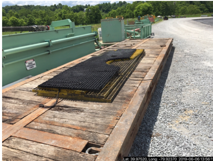
Photo # 6. A section of heavily contaminated grating was found stored off containment on the southern side of the pad.
