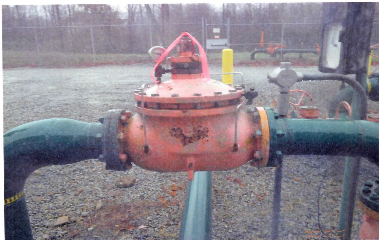
1. Leaking Check Valve Identified with FLIR – LMM Springhill CS – 11/10/2015
